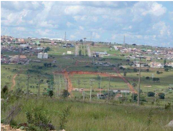
Figure 5-3. Panoramic view of DF-459 under construction
