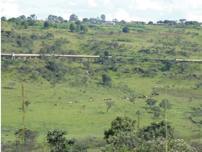
Figure 5-2. Panoramic view of site DF-PA-11 and the above ground sewage pipeline, Condomínio Pôr-do-Sol houses in the back
